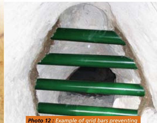
Photo 12 : Example of grid bars preventing access to the cavity.
