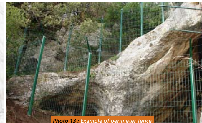
Photo 13 : Example of perimeter fence surrounding the access to cavities.
